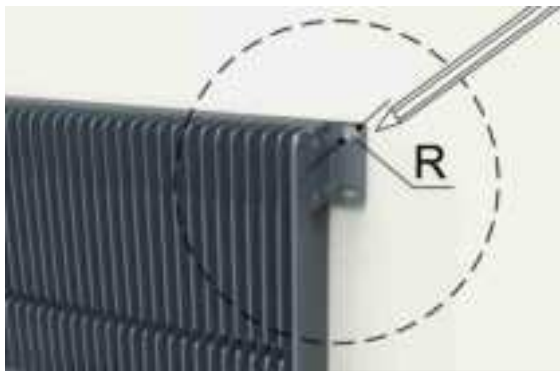
Marking the Position of Mounting Holes
