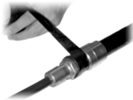
Fig. 8.6-10 Schematic Diagram of Wrapping Waterproof Adhesive Tape (1)
