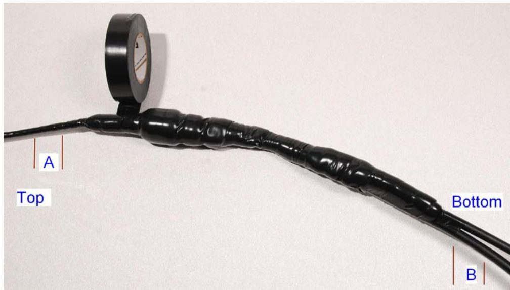
Figure 101 Wrapping PVC tape around the GPS adapter cable joint
