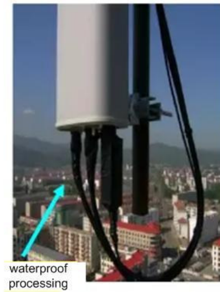
Figure 3-13 Antenna Waterproof Protection
