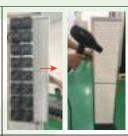
3.Remove dust from the filter with a hair dryer or vacuum cleaner. You can also gently pat the filter.
