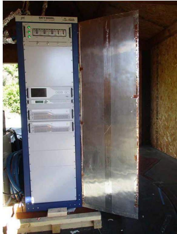
Copper Tape on Aluminum Door
