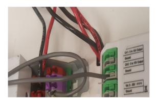
Step 2, Insert red 24vdc wire
