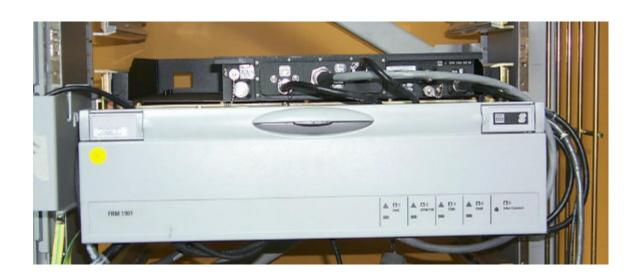
Nortel Networks MFRM Assembly Front View Fan Assembly Mounted
