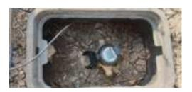
**Step 2)**Remove threaded locking mechanism
