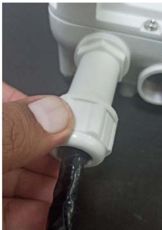
Figure 148: Fitting the gland nut to the rubber seal
