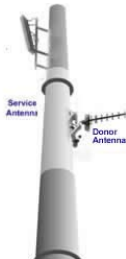
Figure 2-1. Service above Donor Antenna
