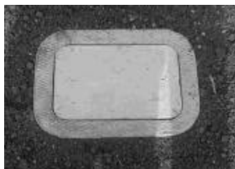
Concrete pit with concrete cover and no lid
