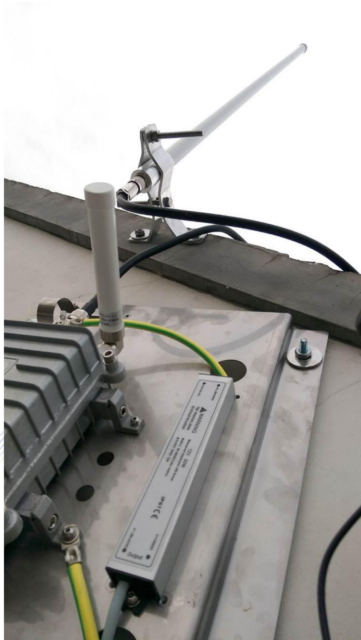
Figure 10 Antenna extension cable installation
