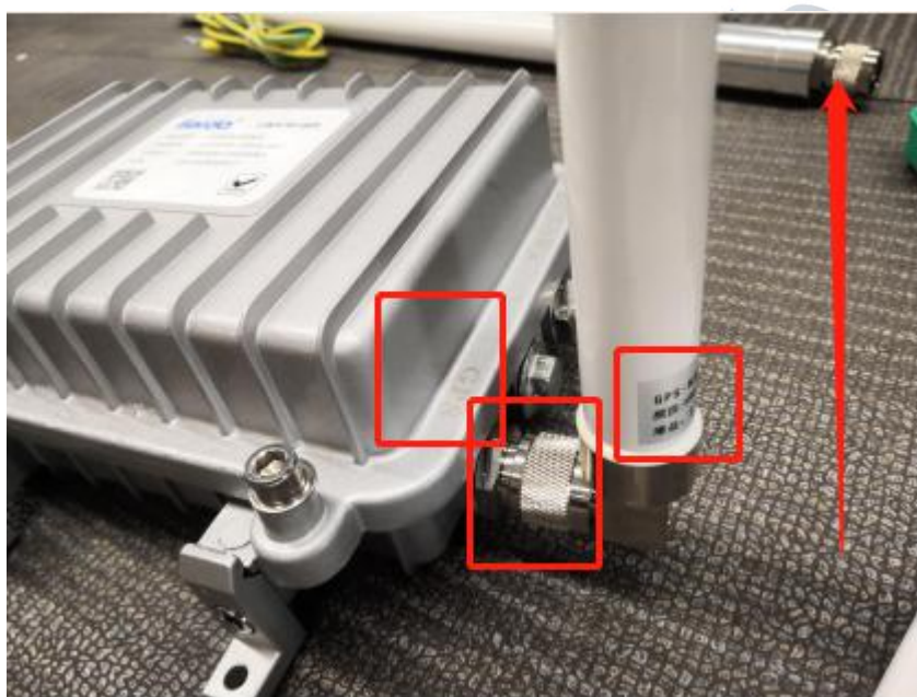
Figure 3 GPS antenna installation
