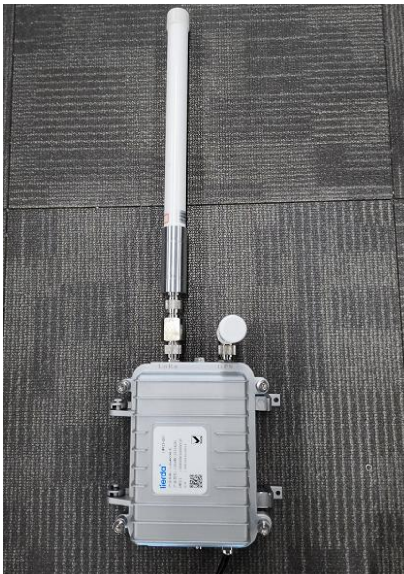
Figure 5 Antenna installation completion display
