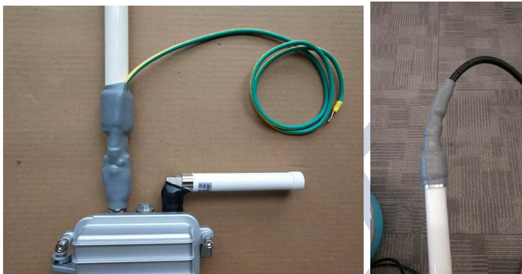
Figure 11 interface waterproofing installation
