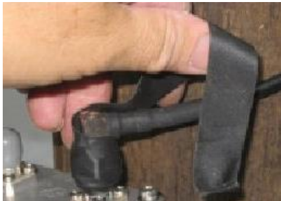
Figure 63: Weather-proof the connection
