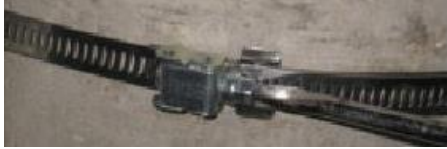
Figure 28: Tighten clamp bands
