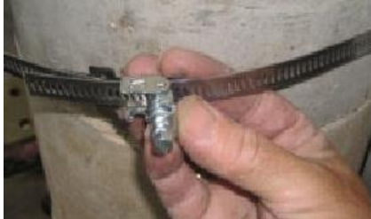
Figure 26: Assemble clamp bands (2 required)
