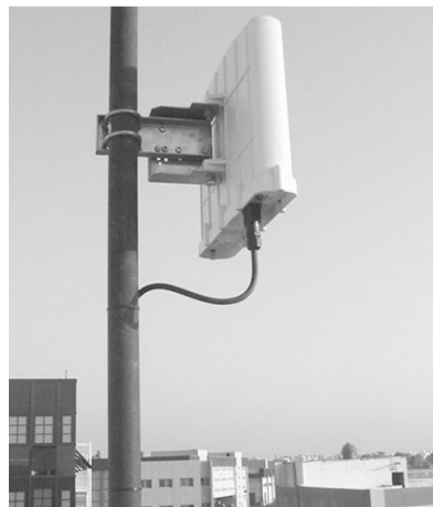
Figure 7-2: Pole-mounted BSR
