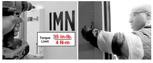
Do not over-tighten the fastener. Do not tighten fastener beyond 35 in-lb. (4N-m).
