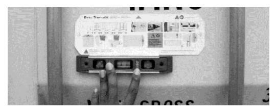
3. Using a drill bit, drill a hole through each of the cross hairs on the template. This will create two holes you will use to mount the module.
