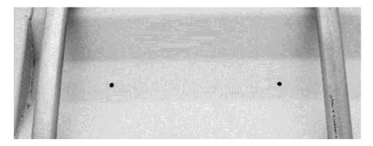
2. Source a set of nylon, rubber, or metal plugs, of the appropriate diameter, to fill the holes. These plugs can be sourced from hardware or auto supply stores. Insert the plugs into the holes. If desired, you may add 100% Silicone Exterior Grade caulk to the rear of the plug for extra protection to seal any gaps against water entry.
