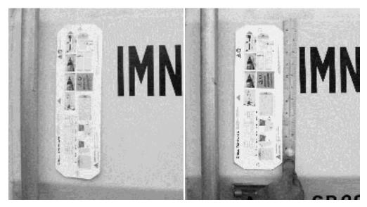
**Technique 2:** Visually, place the template in the desired installation location. Using a level, check that the template is level.
