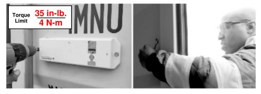
Do not over-tighten the fastener. Do not tighten fastener beyond 35 in-lb. (4N-m).
