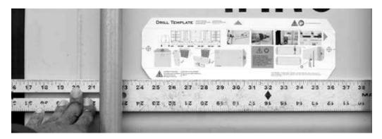
**Technique 2:** Visually, place the template in the desired installation location. Using a level, check that the template is level.
