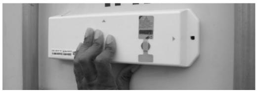
6. Insert your fastener of choice into the holes and use the appropriate tools to secure the module to the asset.
