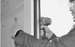
Do not over-tighten the fastener. Do not tighten fastener beyond 35 in-lb. (4N-m).
