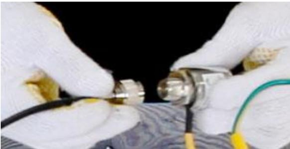
3. The connection point of RF cable needs to be weatherproofed. For more detail, refer to 3.5 Weatherproof Protection. After weatherproof protection, it is shown in Figure 4-5.
