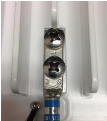
Figure 4: Standard 2 Hole Grounding Lug (2 X M6)
