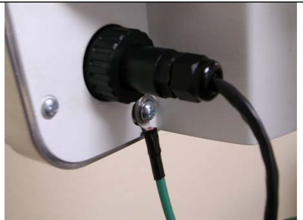
ODU connection ready with ground wire
