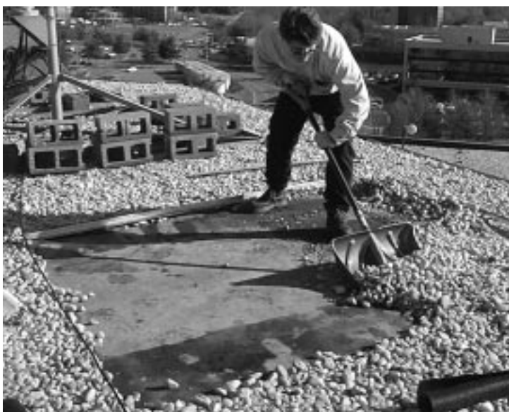
Figure 3-3 Clearing gravel from the installation location
