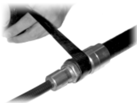
Fig. 8.6-10 Schematic Diagram of Wrapping Waterproof Adhesive Tape (1)
