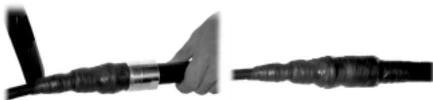
Fig. 8.6-11 Schematic Diagram of Wrapping Waterproof Adhesive Tape (2)
