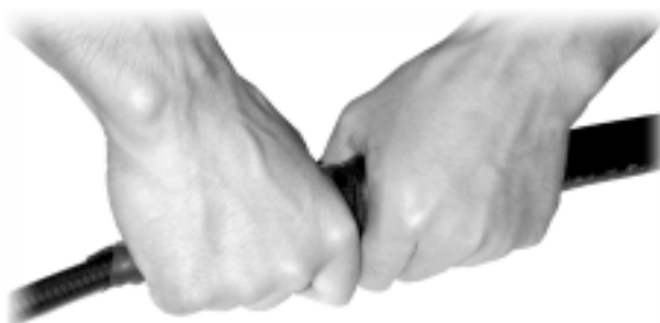
Fig. 8.6-12 Schematic Diagram of Wrapping Waterproof Adhesive Tape (3)
