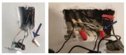
After turning off your breaker, pull out the switches (**WARNING:** there may be multiple circuits in one gang-box -- please ensure all circuits are turned off). Check the back of your gang-box for a bundle of white wires. These are typically neutrals.
