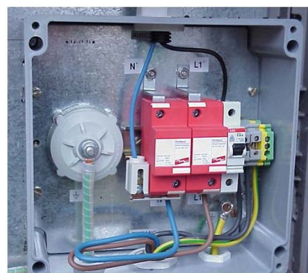
Figure 2-1. Protective Device Installed in Connection with the Power Supply
