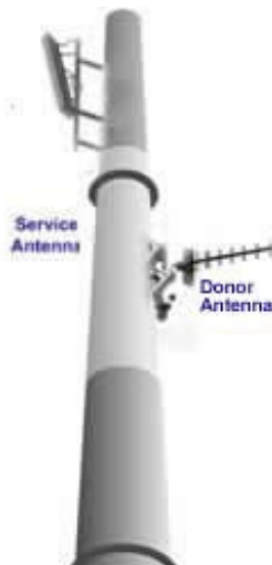
Figure 2-1. Service above Donor Antenna
