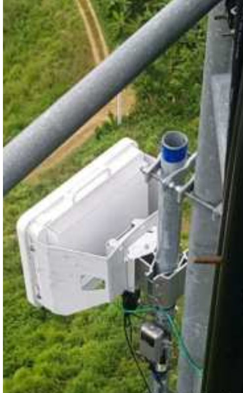
BN Installed on Tower
