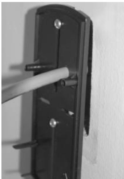
Figure 6> Installing back plate to the wall
