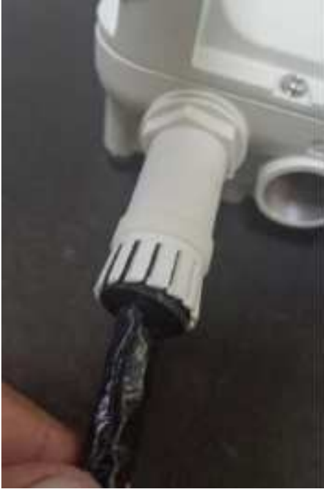
Figure 146: Fitting the gland body
