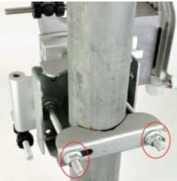
Figure 91: Attaching the precision bracket
