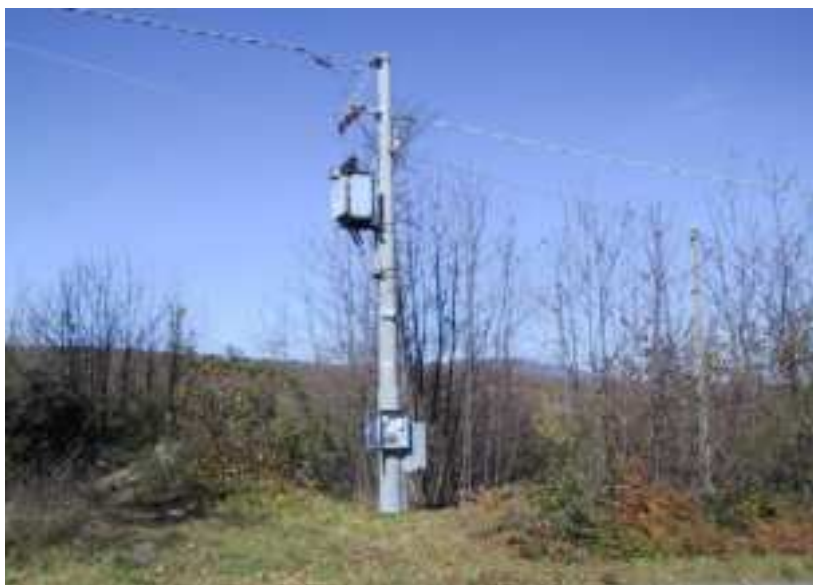
Figure 3 Pole-mounted transformer
