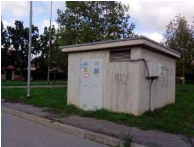
Figure 2 - Pre-assembled substations
