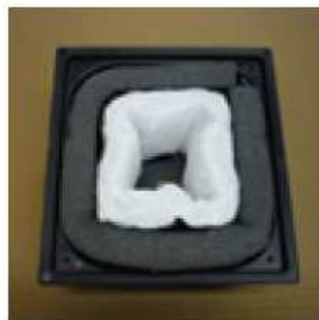
Fig.2 Install 3M foam and acoustic insulation.
