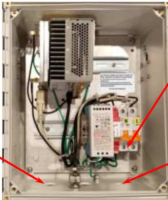
Install AC wiring per label. Ground to an available location on the busbar, Line (black) to “L”, Neutral (white) to “N” terminals.
