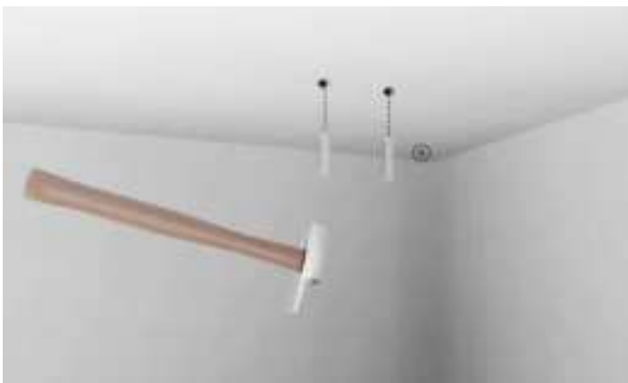
Figure 50. Insert Plastic Wall Plugs
