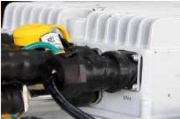
Figure 4-15 Connect the PWR Interface
