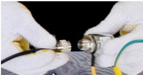
Figure 4-4 Connect the GPS RF Cable to the GPS Lightning Arrestor
