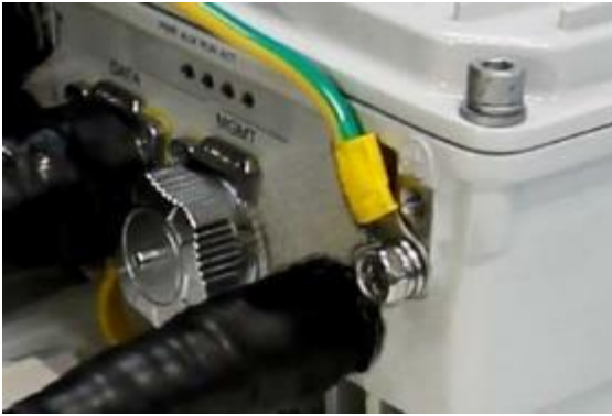
Figure 4-17 Connect GPS Lightning Arrestor Grounding Cable
