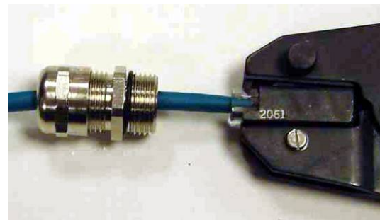
Step 4: Insert conductors and crimp
