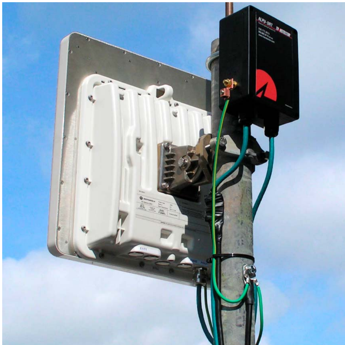
Figure 77 - Upper Grounding Configuration
