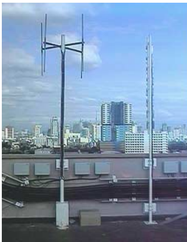
Figure 5-8: Outdoor 10mW RPs installed on rooftop
