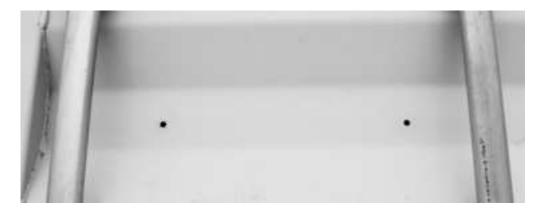
2. Source a set of hylon or rubber plugs, of the appropriate diameter, to fill the holes. These plugs can be sourced from hardware or auto supply stores. Insert the plugs into the holes. If desired, you may add 100% Silicone Exterior Grade caulk to the rear of the plug for extra protection to seal any gaps against water entry.
