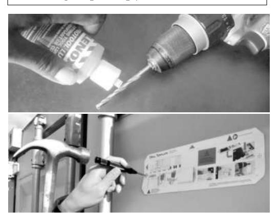
4. Remove the template. You now have two holes in the door. If there are any burns around the holes, remove them at this time. Also, remove any dust or debris left over from the drilling or de-burring operations and ensure surface is clean and dry.
