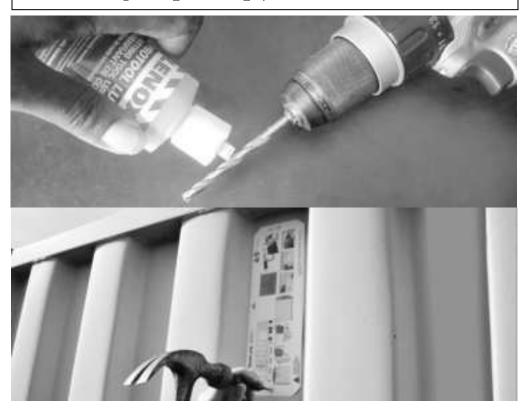
4. Remove the template. You now have two holes in the container. If there are any burrs. around the holes, remove them at this time. Also, remove any dust or debris left over from the drilling or de-burring operations and ensure surface is clean and dry.
