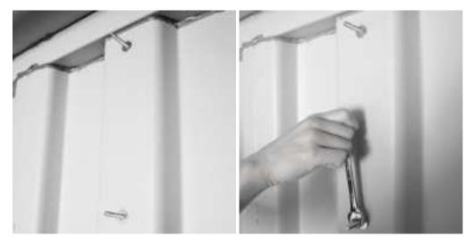
Tip: If, when installing the nut on the carriage bolt, the carriage bolt becomes dislodged from the module, you may complete the installation of the nut by grasping. the threads of the bolt with a set of pliers, pulling the bolt to reset the square neck into the booket and tightening the nut with a wrench.
