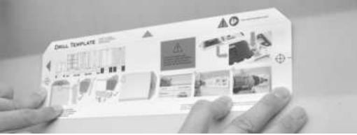
Tip: If you are planning to install the module inside of a corrugated feature, where the rear surface of the feature is narrower than the template, you may fold the upper and lower ends of the template along the perforations
