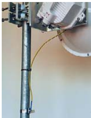
Fig. 4.10: Grounding the RAY unit
