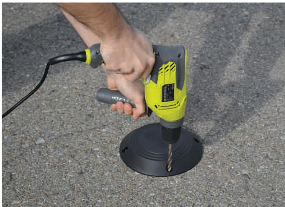
*Figure : Indicating the holes for the node*
