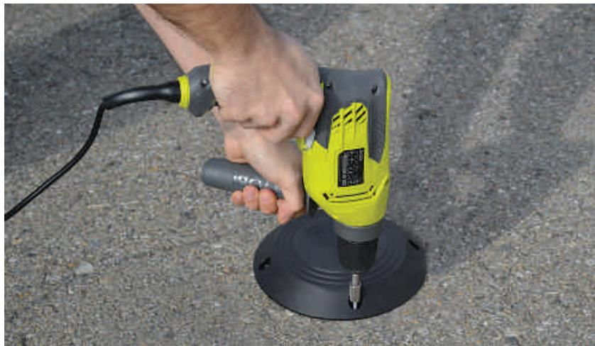
Figure : Screwing the node
