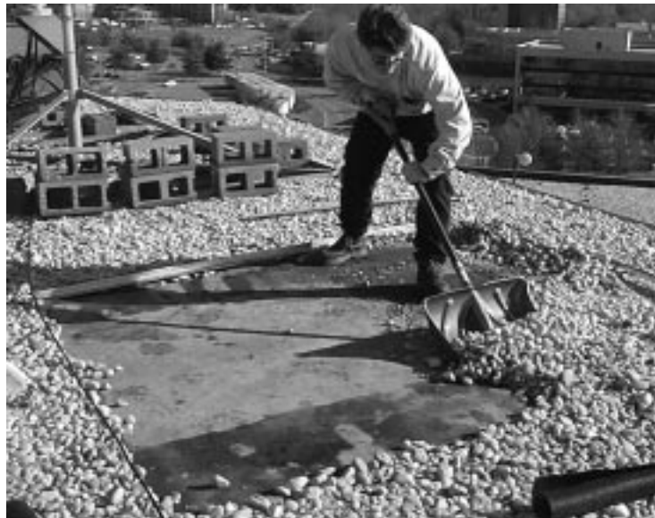
Figure 5-2 Clearing gravel from the installation location
