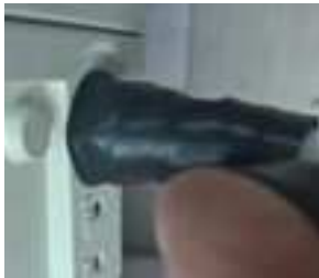
Figure 12: Weather-proof the CRTV RF Connection
