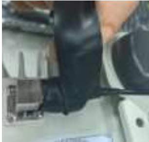
Figure 9: Weather-proof the GPS Connection
