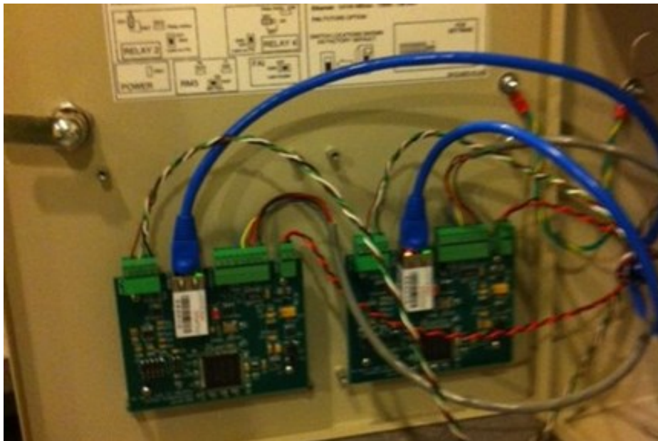
Two reader control panel configured with EWACs (each reader requires an EWAC board). Note, Power connections and those to the panel are shown here.
