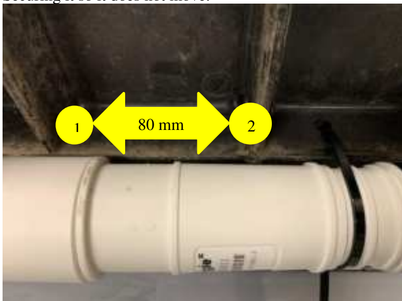
Figure 4: Drill hole spacing
