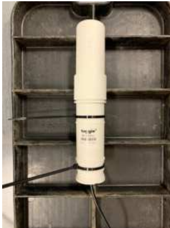
Figure 5: Trim excess cable ties length and discard appropriately
