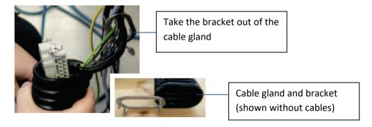
Fig. 53: Take the bracket out of the cable gland
