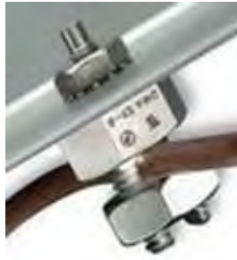
Figure 4: Detail of the grounding screw.
