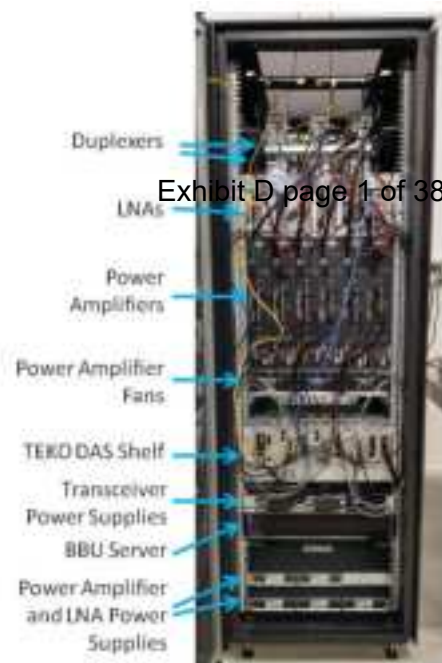
Figure 2: 900 MHz eNodeB Rack Components
