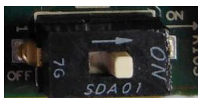
Figure 6 – SBC Switch (SW2)
