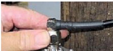
Figure 10: Connecting Antenna RF Cable
