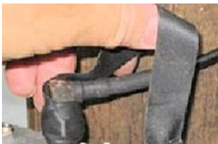
Figure 11: Weather-proof the Connection
