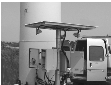
Figure 4-1: Example of a sun shield
