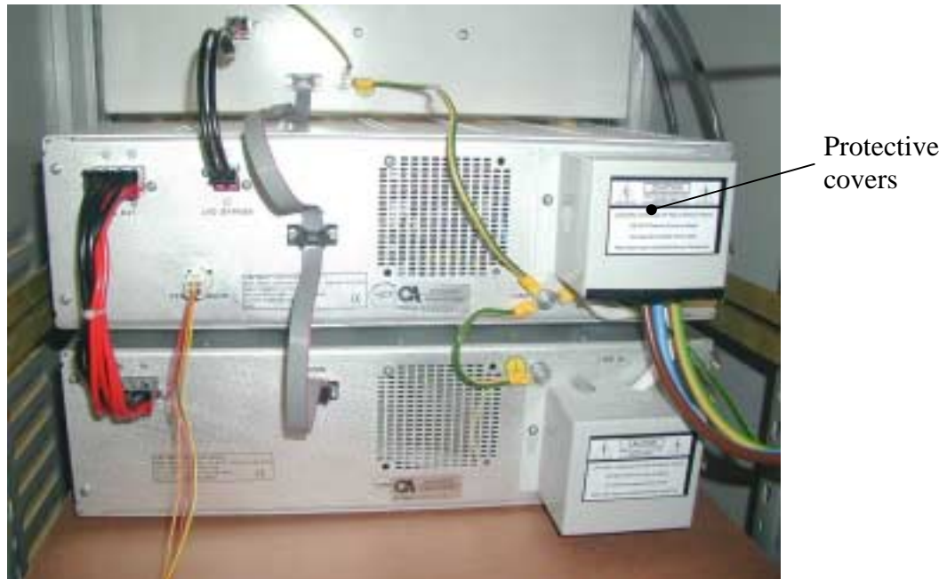
Figure 7-7: Rear BSPS cable connections
