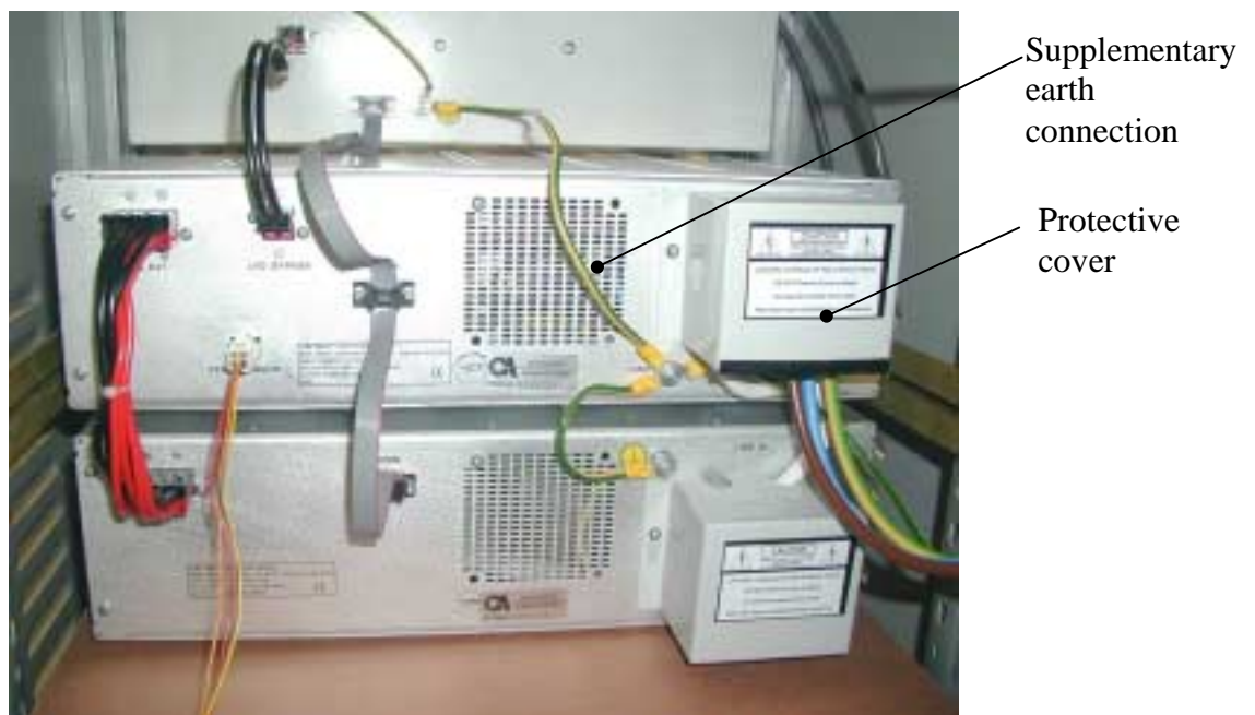
Figure 7-15: Fitting protective covers over terminal block
