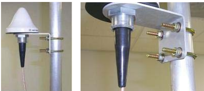
Figure 43 GPS antenna mounting
