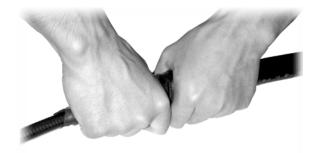
Fig. 10.6-3 Wrapping the Waterproof Adhesive Tapes (3)
