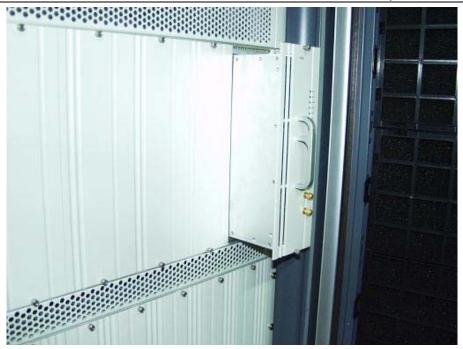
Fig. 12.3-3 Loosening the Screws and Unplugging the RFE
