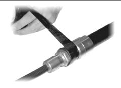
Fig. 10.6-1 Wrapping the Waterproof Adhesive Tapes (1)
