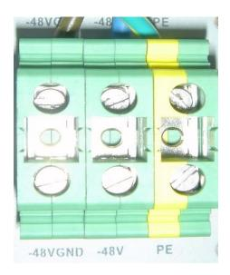
Fig. 5.1-1 BDS Power Cable Installation on BTSB
